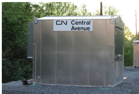
New PTC control shack on the P&I
