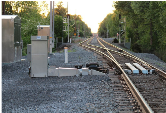
New switch heater at Central Ave on the P&I at Paducah
