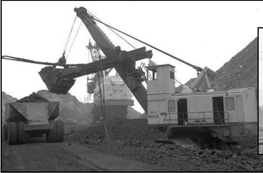
A Marion electric shovel loads coal in the foreground while in the background a larger crane strips away the overburden. 1959, Cliff Downey collection
