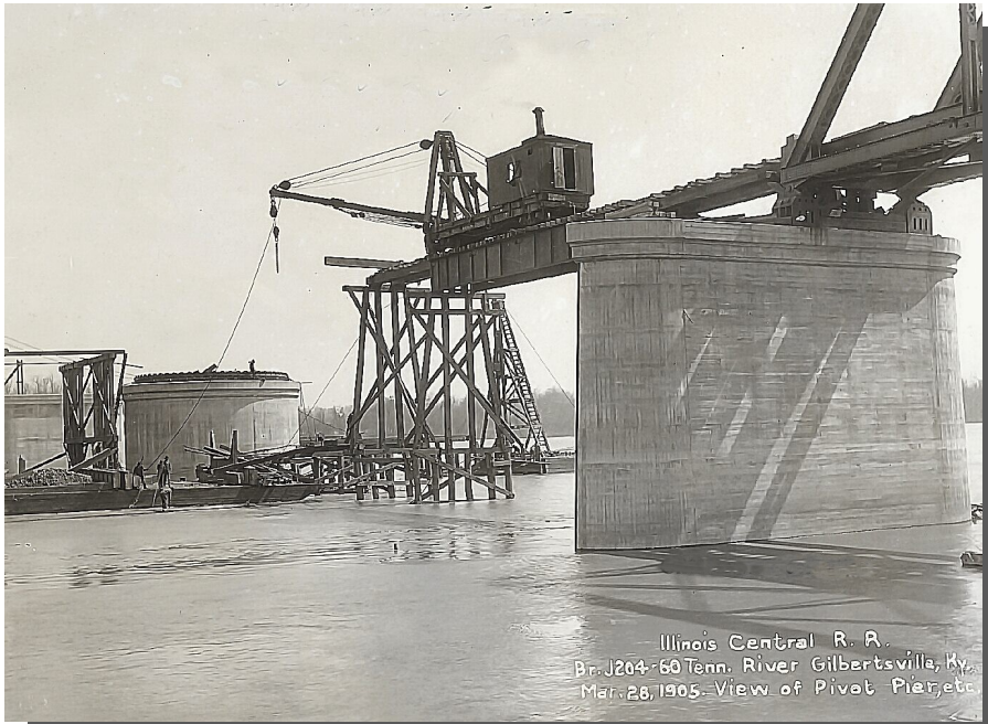
Construction of the IC swing bridge on the Tennessee River 1906 Note the large pivot for the bridge. From the Cliff Downey Collection
