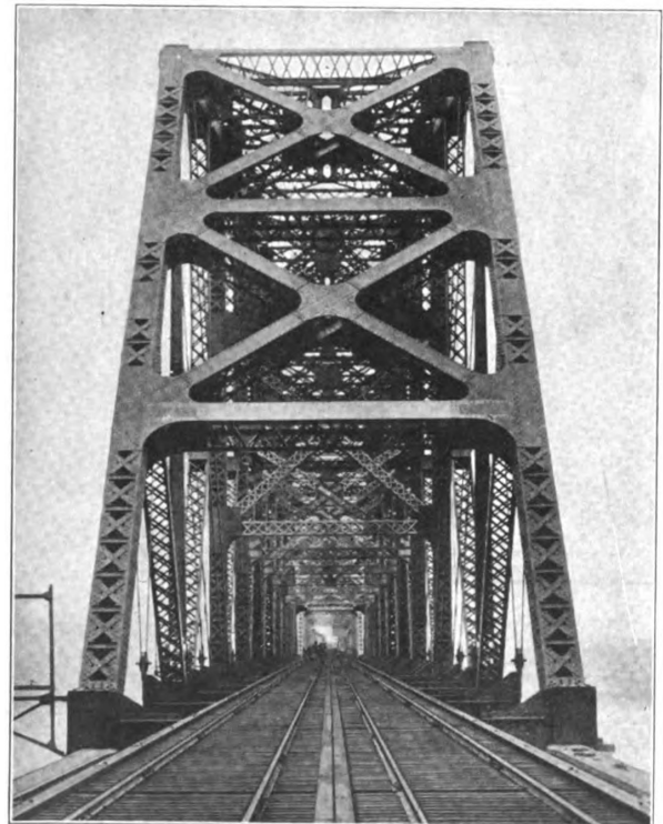
1918 End view of the bridge. The double track shown was artist rendition as the engineer reported only one track was constructed. The entire P&I infrastructure was made for double track but never completed. This evidence can be seen at bridges crossing 32nd street, Jefferson and Broadway streets in Paducah
