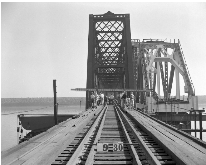
This photo was taken at 9:30am, shortly after crews began moving the first new span of the Cairo bridge. Yes, that is a giant yardstick in the distance. It was used to measure movement of the two spans. IC photos, Cliff Downey collection
