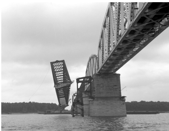
By 1:29pm the first span to be replaced on IC's Cairo bridge was completely out of the way. Crews will soon begin moving in the new span. IC photo. Cliff Downey collection.
