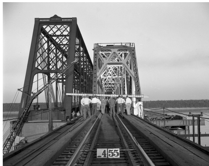
By 4:55pm the new span was almost in place. Once movement is complete, crews will begin reconnecting the rails, signal wires, company telephone, etc., and the bridge will reopen shortly after midnight. IC photo, Cliff Downey collection.
