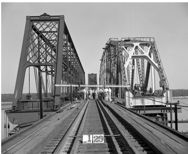
By 1:29pm the first span to be replaced on IC's Cairo bridge was completely out of the way. Crews will soon begin moving in the new span. IC photo. Cliff Downey collection.
